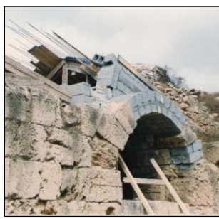
Figure 11: Using concrete and reinforcement steel in the roof of the eastern entrance of the theatre[10].
