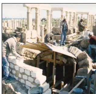
Figure 12: Using the limestone bricks to roof the western entrance of the theatre [10].
