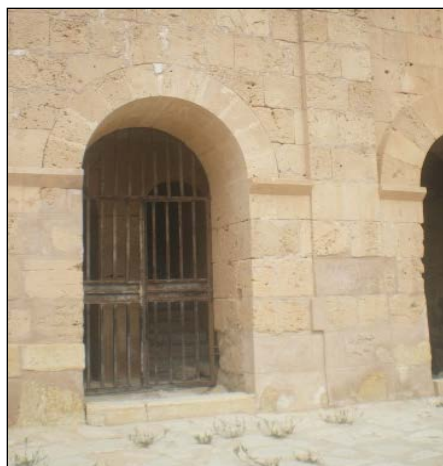
Figure 5: Treatment of arcs using materials of the same original building material [5].
