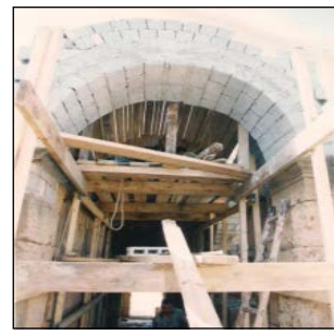
Figure 10: Using the cement block in the theatre [10].
