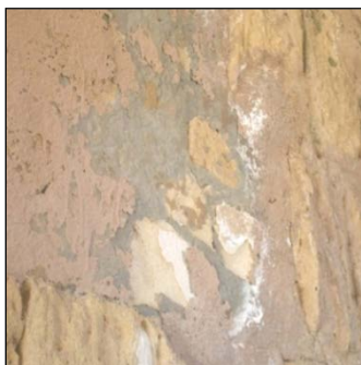
Figure 9: The use of black cement and paint it with a contemporary paint,(Authors,2012)
