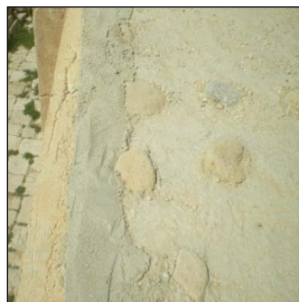
Figure 8: Using concrete in the floors and surfaces,(Authors,2012)
